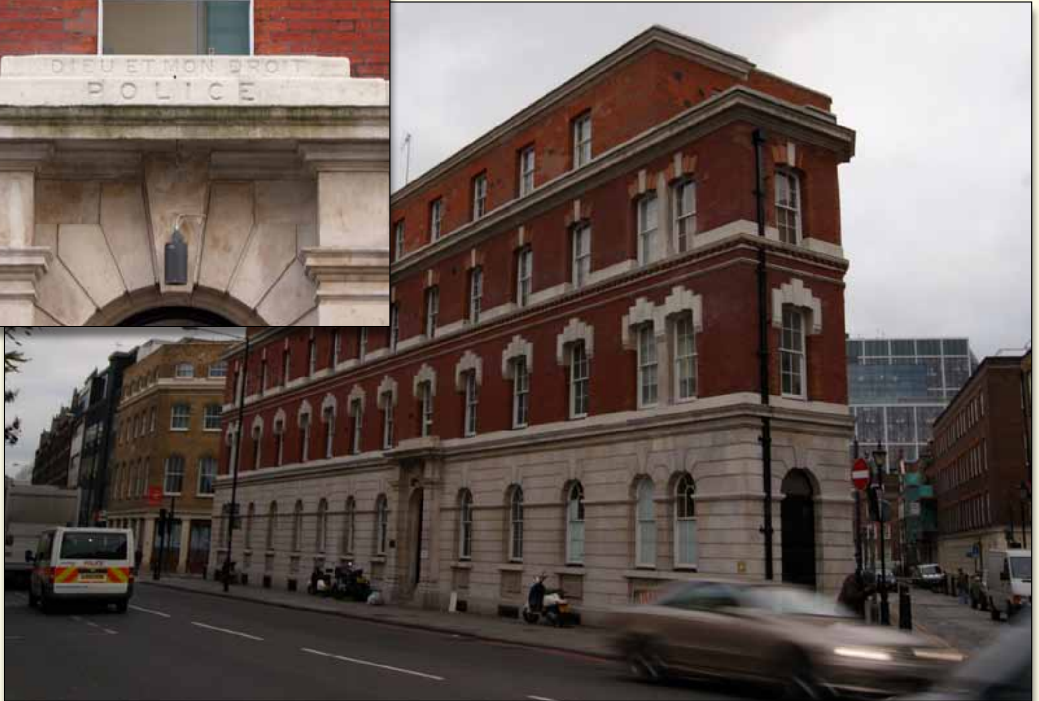
COMMERCIAL STREET POLICE STATION 2010 (INSET SHOWS DOOR DETAIL)
