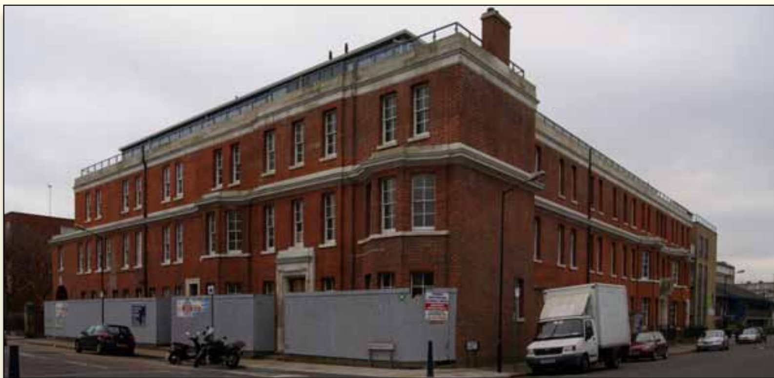
ARBOUR SQUARE POLICE STATION & THAMES POLICE COURT 2010
